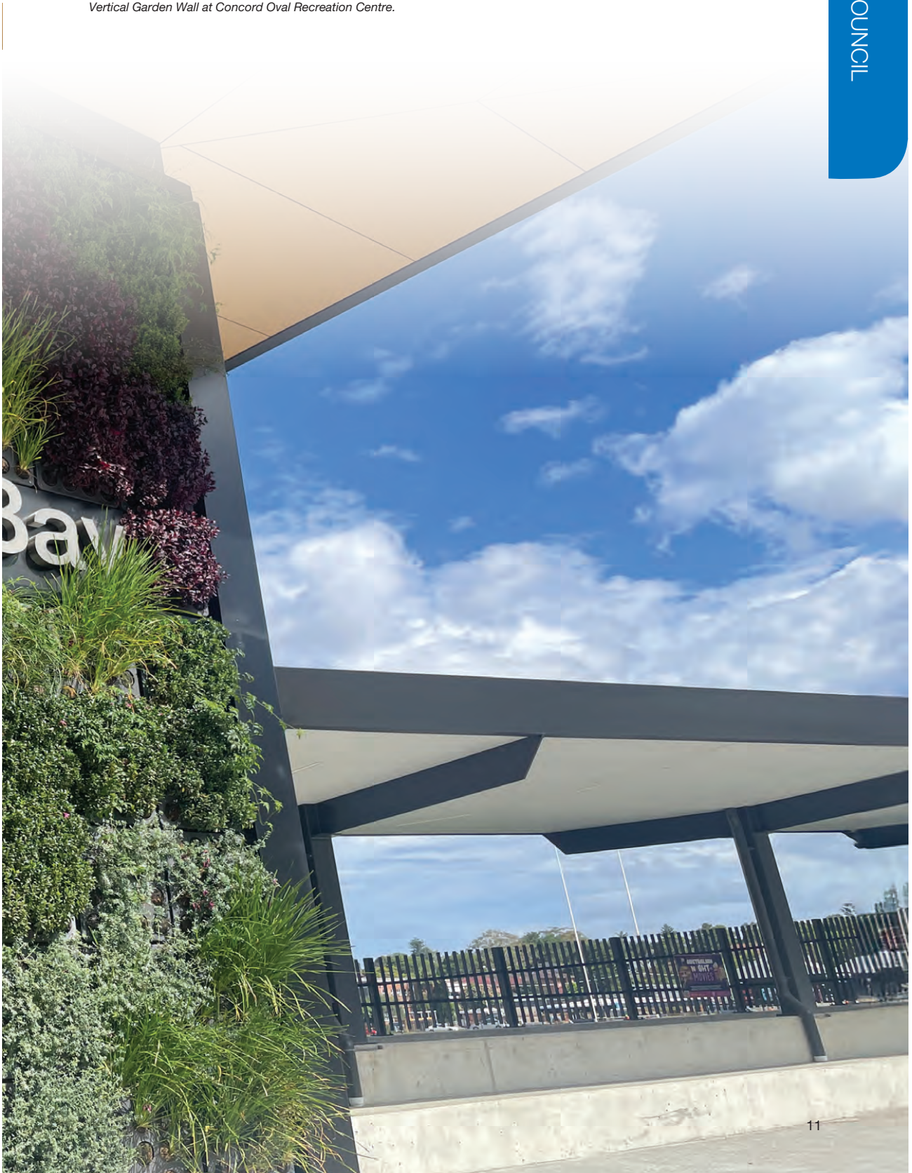
Vertical Garden Wall at Concord Oval Recreation Centre.
