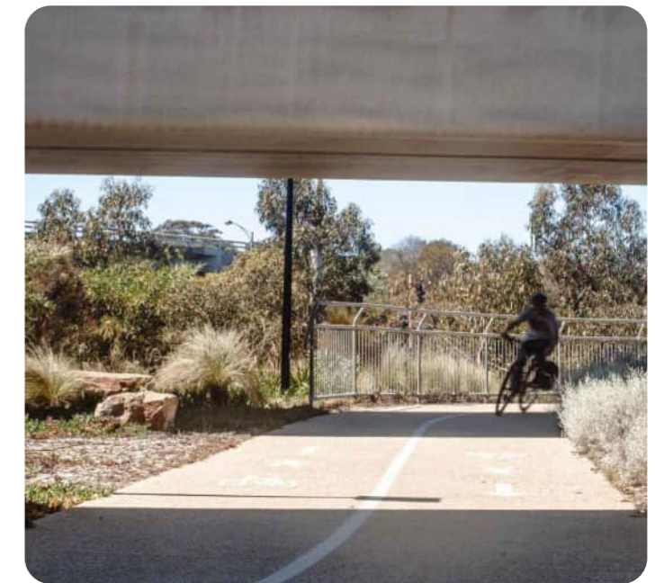
Shared path under bridge (Skye Road. Source: Tract)
