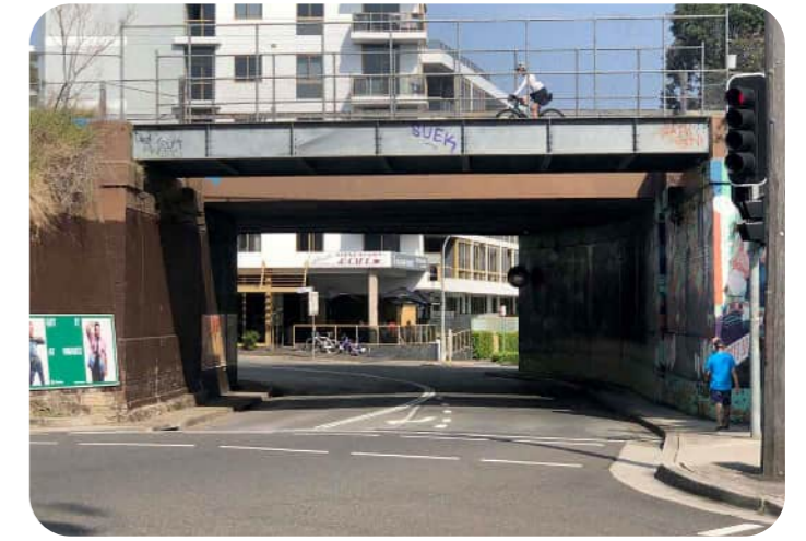
Inefficient width of pedestrian/cycling link under railway bridge
