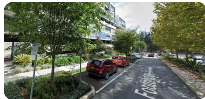
Tree planting blisters, Footbridge Bvd, Wentworth Point (Source: Google Maps)
