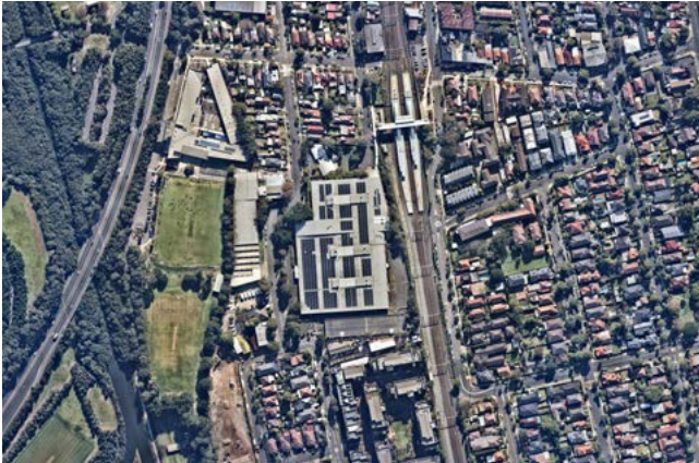
Figure K24-1 Aerial photo (source: nearmap.com)
