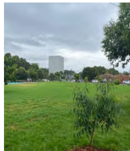
Figure 17: M4 Ventilation Shaft as viewed from Arnotts Reserve
