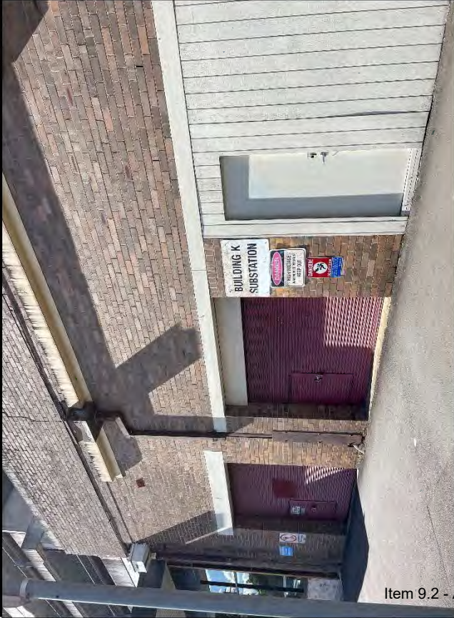
PHOTO 93: BAKEHOUSE QUARTER, AREA 2, SUBSTATION ON GEORGE STREET
