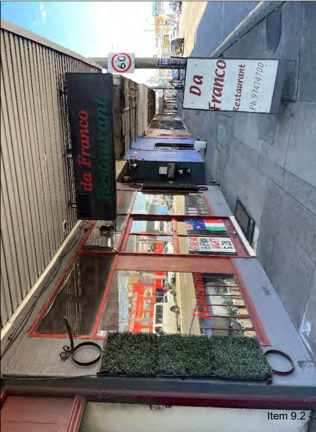
PHOTO 57: WEST BURWOOD, AREA 2, RESTAURANT STOREFRONT ON PARRAMATTA ROAD
