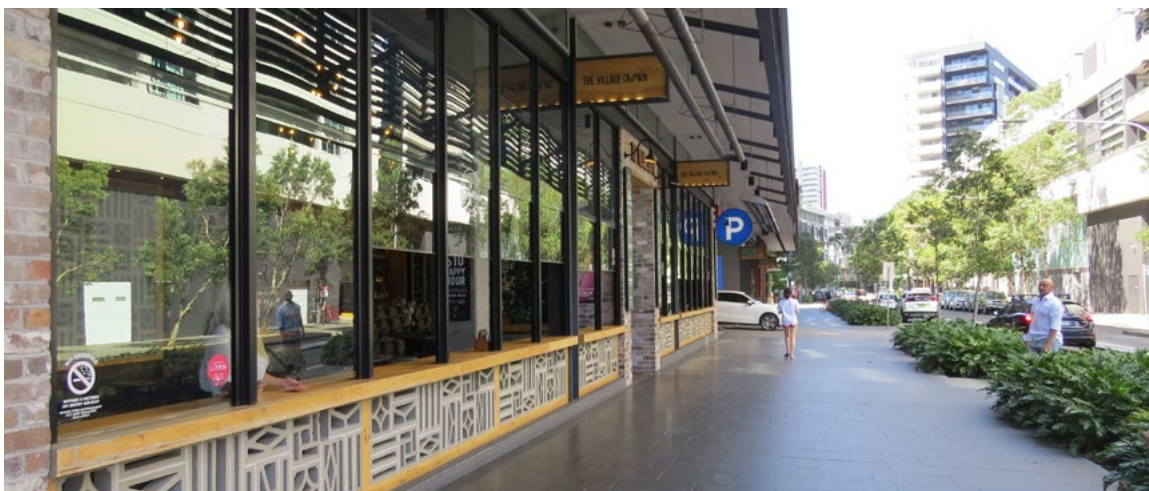
Stall risers, richness of material choices and operable glazing contribute to high quality street interfaces
