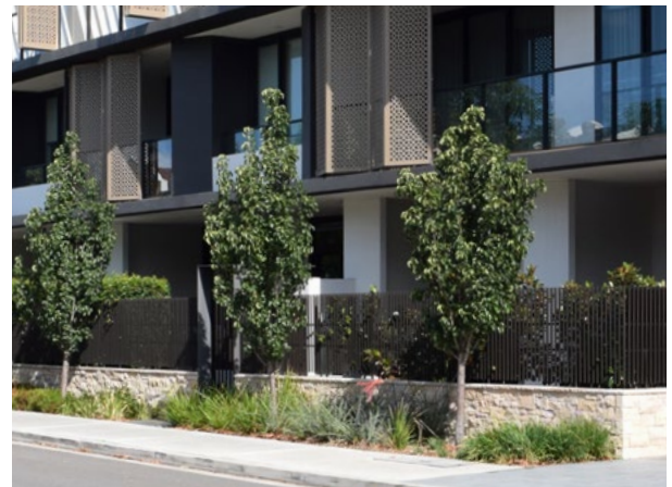
A low stone wall and visually permeable fencing provides privacy for ground floor units and passive surveillance of the street.
