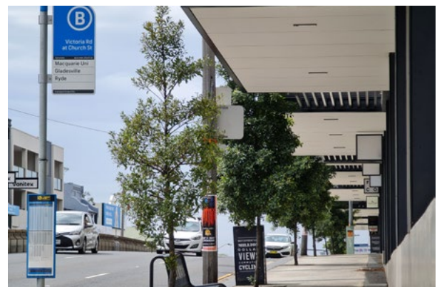
Figure K21-41 Awnings should be designed to allow for street tree planting
