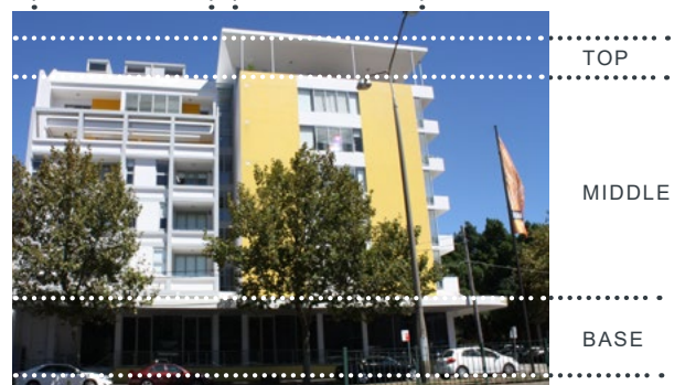
Example of a building that is vertically articulated into two components and differentiates between base, middle and top
