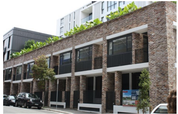
Contemporary use of face brickwork
