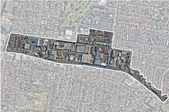
Figure K20-2 Aerial photo (source: nearmap.com)
