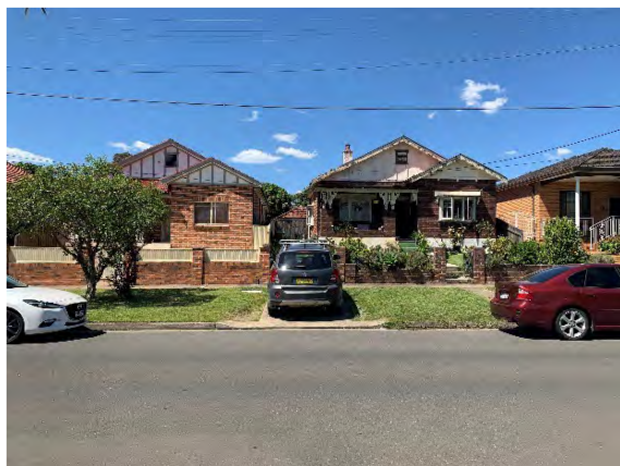
Figure 4.5 Taylor Street, east side.
