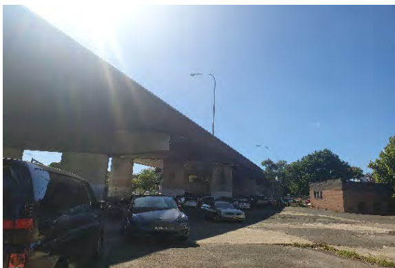
Figure 4.21 Western Motorway overpass.
