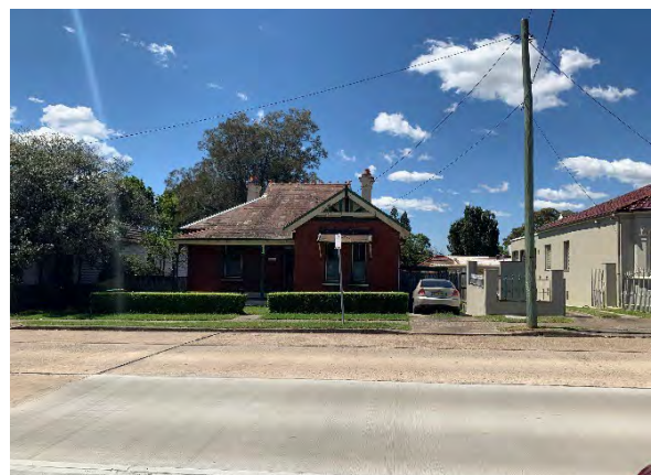
Figure 2.13 House, 33 Burwood Road (#147).
