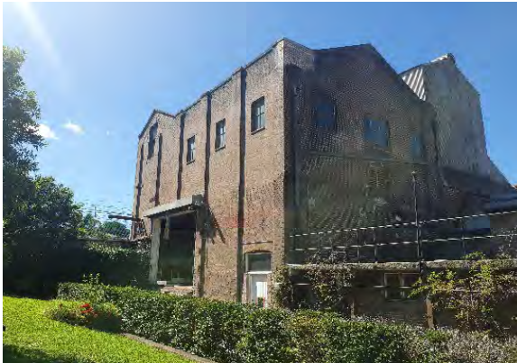
Figure 2.26 Former Arnott's factory.
