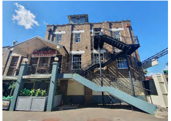
Figure 2.27 Former Arnott's factory.
