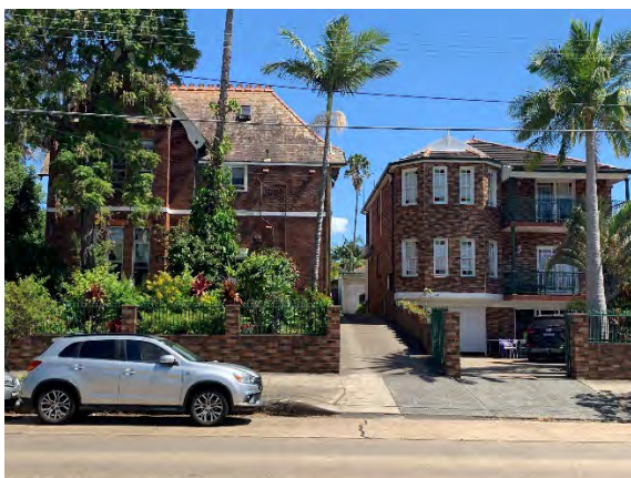
Figure 2.12 Anglican Rectory, 24 Burwood Road (#146), and sandstone kerbing at 22–26 Burwood Road (#155).
